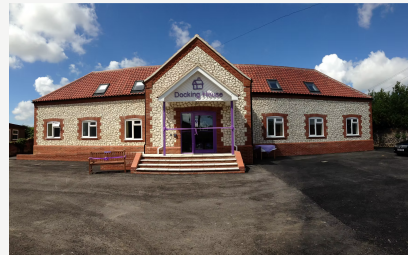
DOCKING HOUSE DEMENTIA CARE HUB
